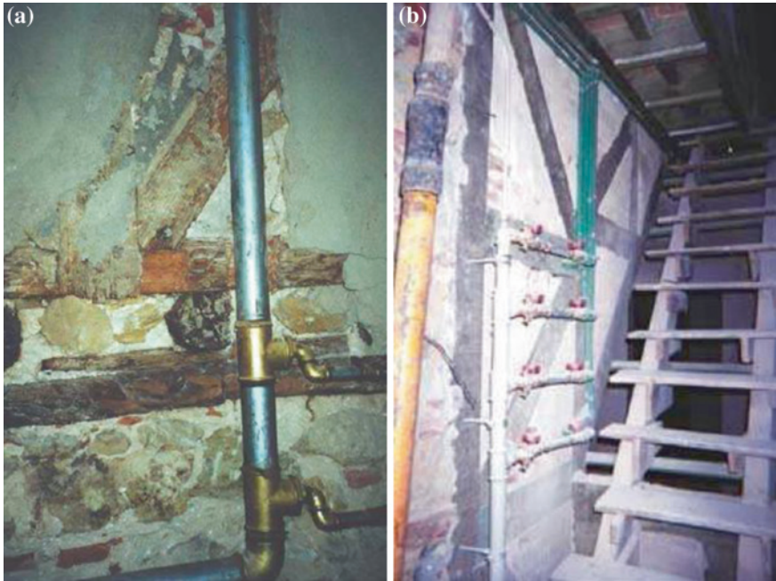
Fig. 20 a Cut in frontal wall to introduce pipes and b pipes crossing wall in the perpendicular direction [20]
