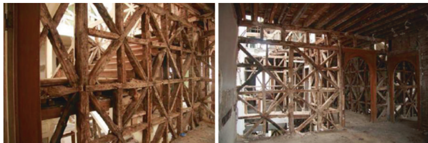
Fig. 1 Gaiola after removal of cover and masonry
