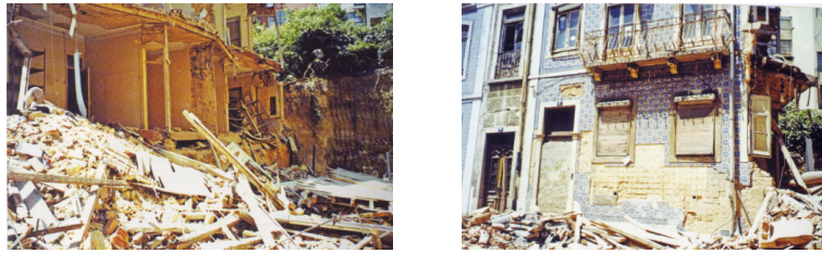
Figure 20 – Collapse of 'Gaioleiro' buildings (Lopes et al. , 2008).
