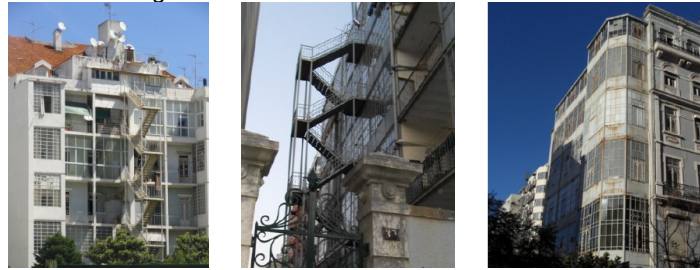
Figure 6 – Metallic service stairs and galleries on 'Gaioleiro' buildings (Andrade, 2011).
