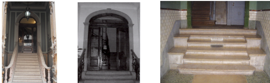
Figure 10 – First flight of masonry staircase gives access to an elevated ground floor with ventilated box underneath (Andrade, 2011 and Appleton, 2005).
