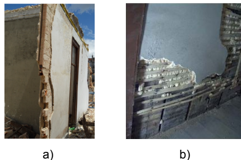
Figure 15 – Interior structure characteristic of 'Gaioleiro' buildings: a) Solid ceramic brick wall (Andrade, 2011); and b) 'Tabique' walls (Pena, 2008).
