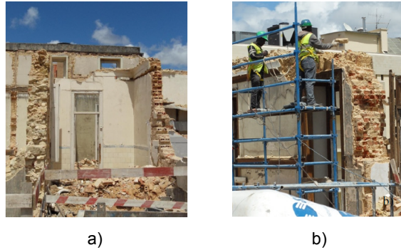
Figure 13 – Brick masonry walls (Andrade, 2011): a) Example of a light-shaft with rubble stone masonry wall (on the left) and solid brick masonry wall (on the right); b) Hollow brick masonry wall.
