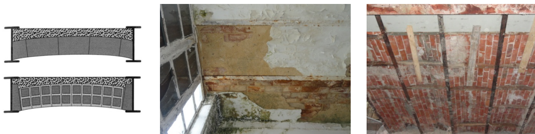
Figure 18 - Floors made of metallic beams and ceramic bricks interconnected by mortar or cement (Appleton, 2005).
